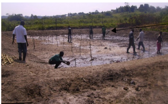
Figure 13: Smoothening and levelling the Pond Bottom. The pond bottom should be sloped towards the outlet. Remember to compact the floor again once done.
