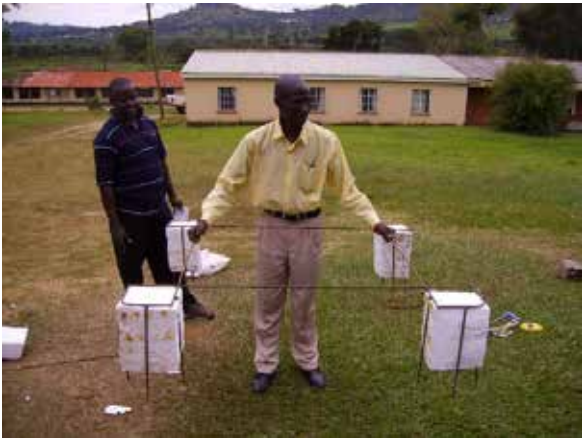
(a) Polystyrene blocks attached to the frame to make a collar. Cover them before installation in water.
