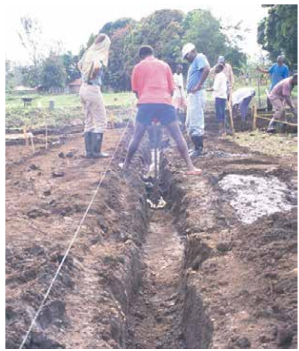
(b) Compact trench with good clay soils. Do not allow the core trench to dry and crack before covering.
