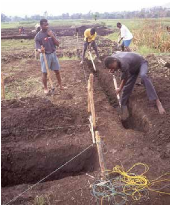
(a) Dig a trench around perimeter pegs. Even a shallow core trench allows root zone to be cut.
