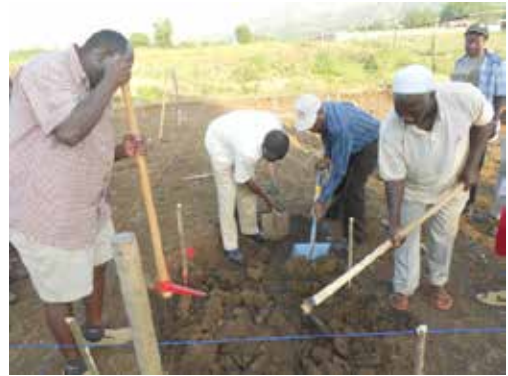
Figure 7: Pegging the pond. (a) The outer line is the perimeter. The central line shows where the inlet pipe and outlet shall be placed. The central line pegs are points at which levels are measured to guide sloping of pond floor towards drainage. The pond floor slope from each corner towards the drainage should be not more than 2%. Note the top soil has been removed and put to the side. It will be used to cover and plant grass on the dyke after construction. (b) The inside toe also needs to be pegged. The outer line (perimeter) forms the centre of the dam wall (more details below)
