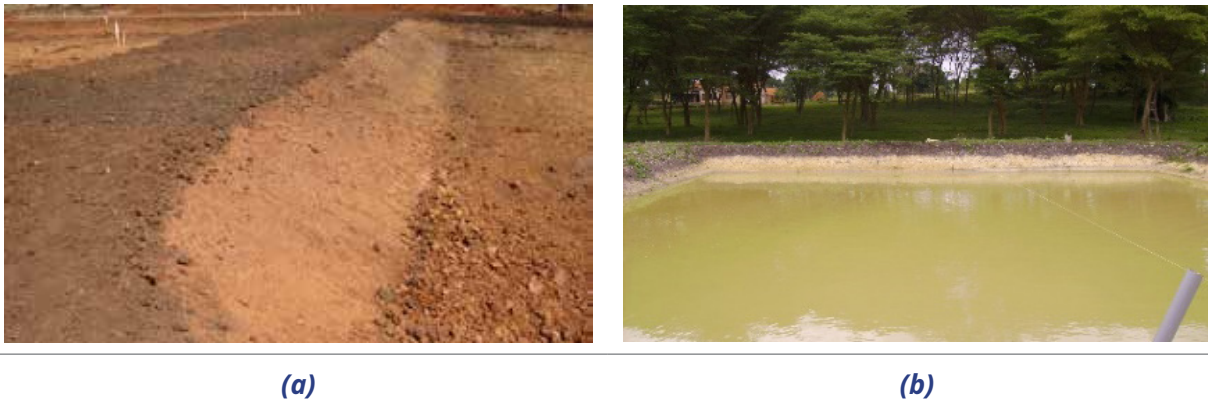
Figure 14: Finishing the Bank.
