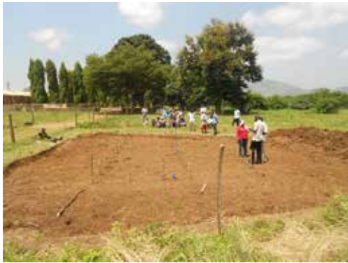
Figure 7: Pegging the pond. (a) The outer line is the perimeter. The central line shows where the inlet pipe and outlet shall be placed. The central line pegs are points at which levels are measured to guide sloping of pond floor towards drainage. The pond floor slope from each corner towards the drainage should be not more than 2%. Note the top soil has been removed and put to the side. It will be used to cover and plant grass on the dyke after construction. (b) The inside toe also needs to be pegged. The outer line (perimeter) forms the centre of the dam wall (more details below)
