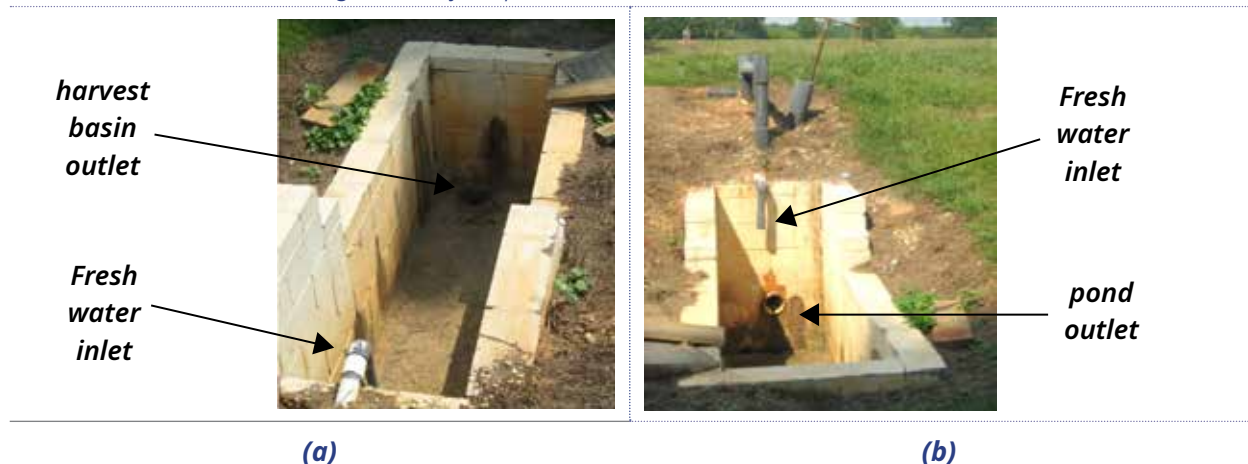
Figure 11: Harvest Basin Outside Pond. (a) View from pond wall showing outlet within harvest basin (b) View showing water inflow points into harvest basin
