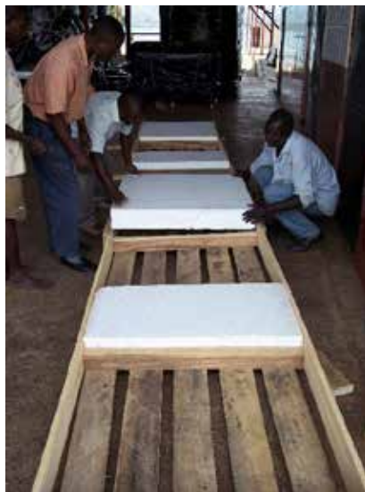
(c) Floating wooden platform
